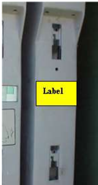
Figure 21 – ABB LV disconnecter label location example.
