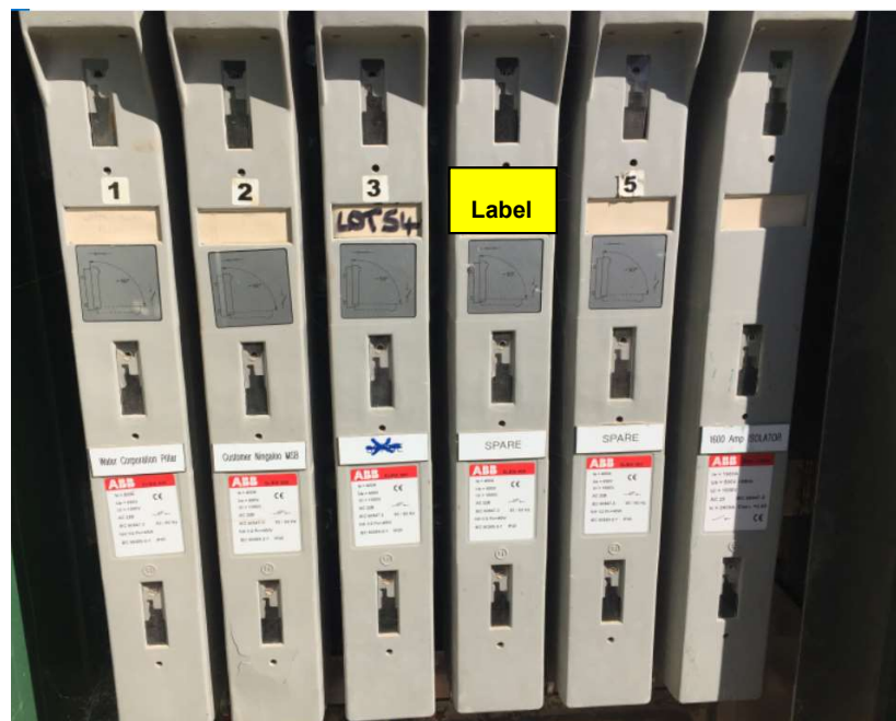
Figure 26 – Pronutec fuse switch example label location.
