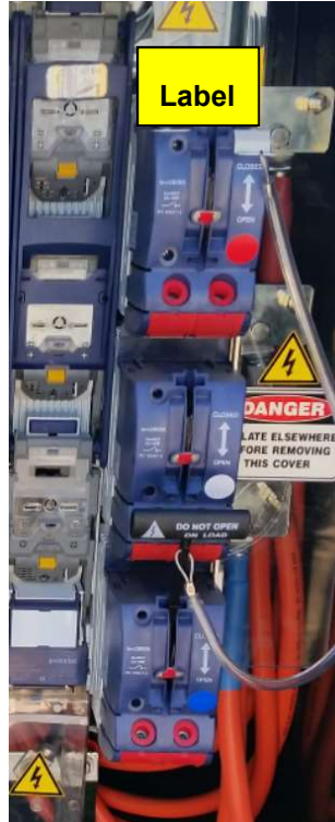
Figure 20 – ABB LV disconnecter label location example.
