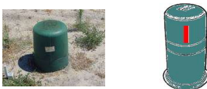
Figure 27 – Universal Pillar with normally-open point with 'I' marking.
