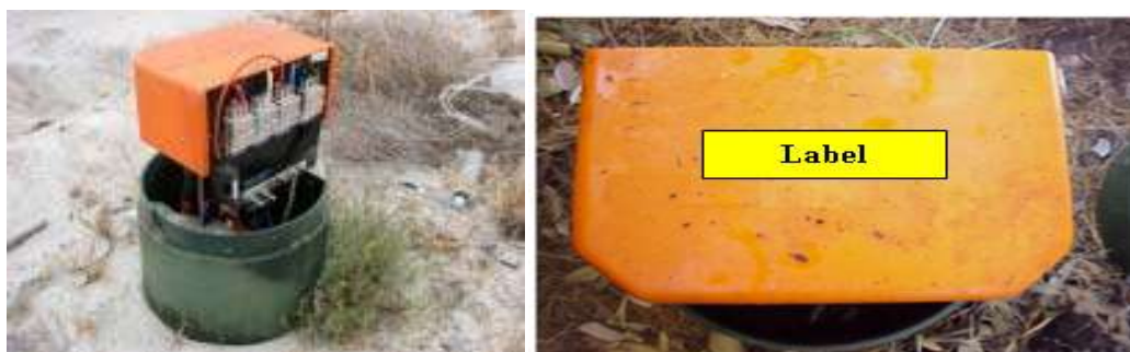
Figure 28 – Universal pillar label location example.
