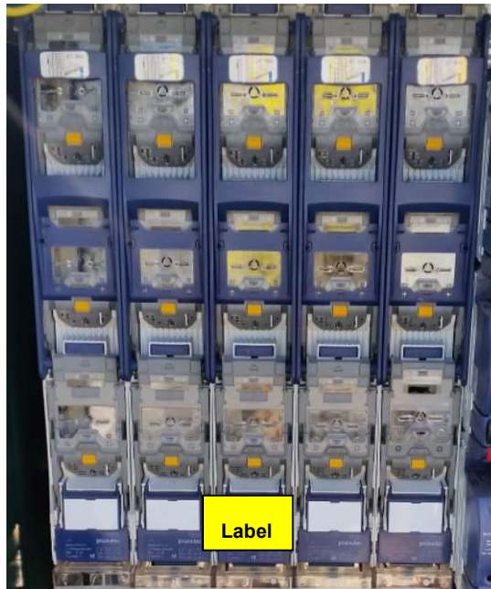
Figure 25 – Pronutec fuse switch example label location.
