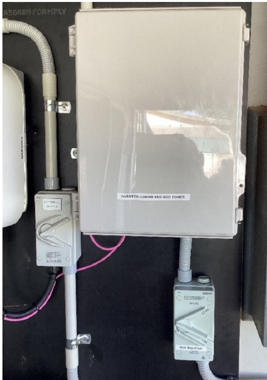
Figure 13: Example SGD enclosure
