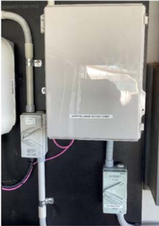
Figure 5: Example SGD installation
