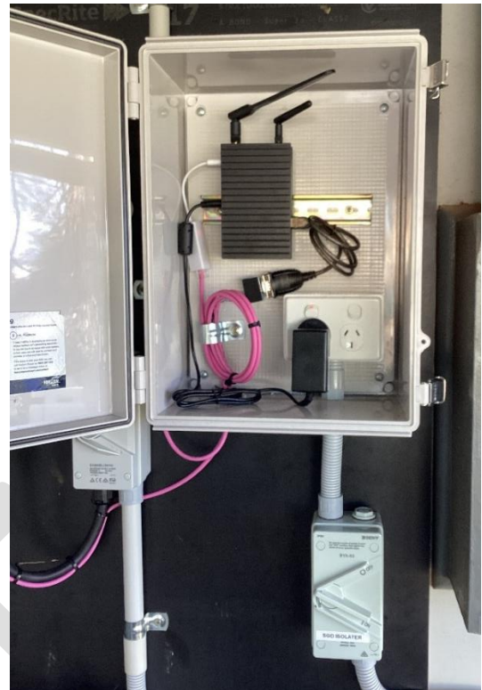
Figure 14: Example SGD enclosure open
