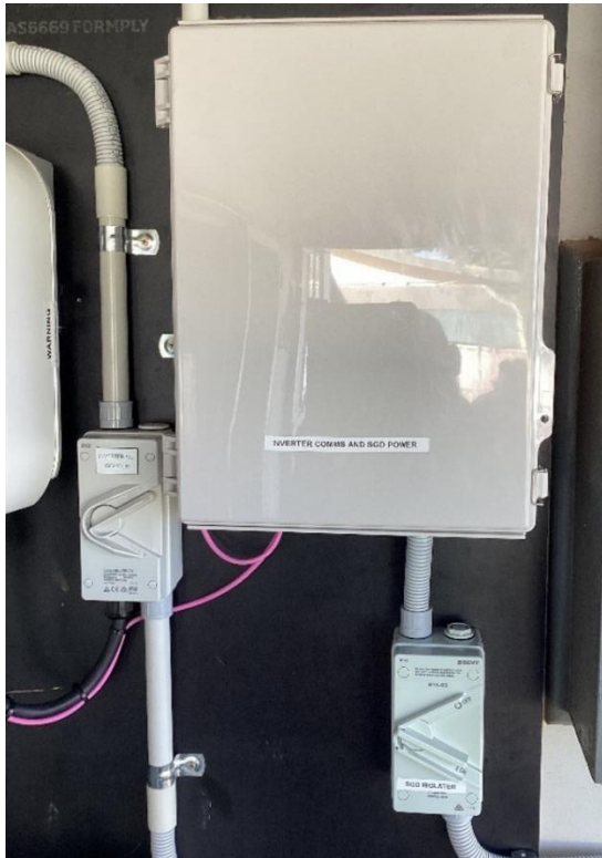
Figure 13: Example SGD enclosure
