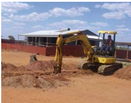
Trenching is underway in Nicholson Camp, Halls Creek
