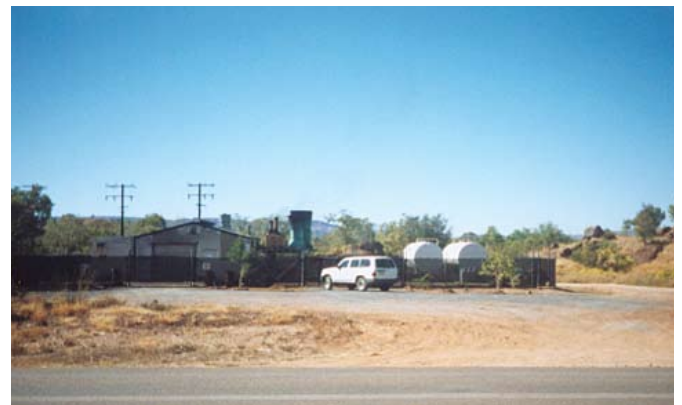
The existing Warmun power station will be replaced with a new, environmentally friendlier power station.
